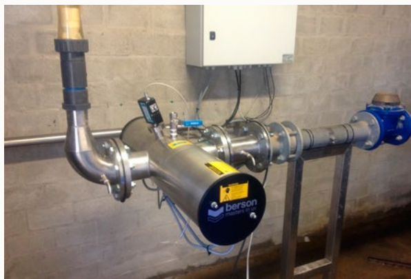
Berson UV system for the treatment of waste water.
